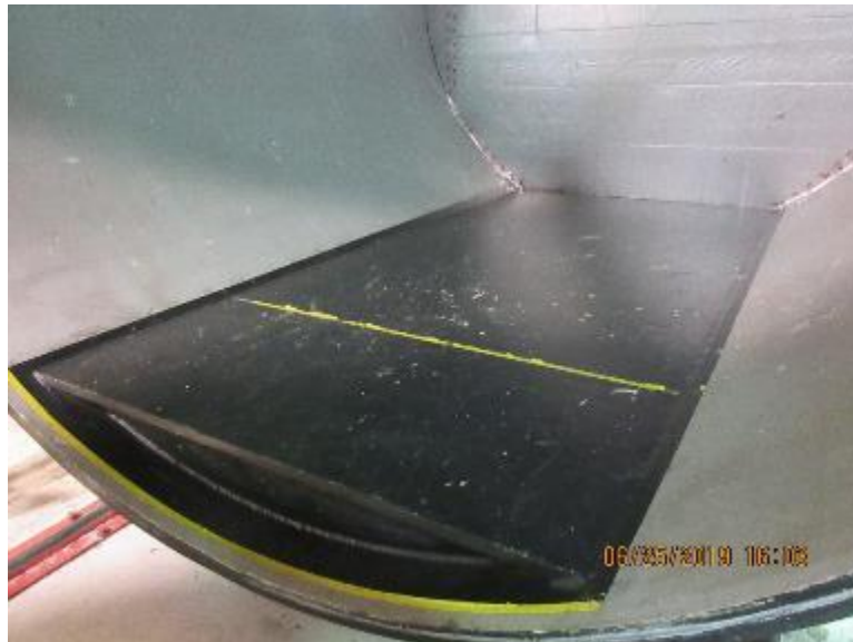
Photo No. 3 Post-test Specimen #1, Witness Chamber
